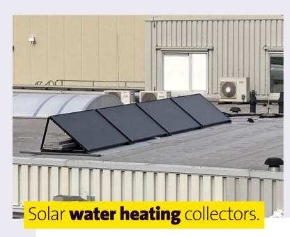
Zeelandia installed four solar water-heating collectors on the roof of its technical department workshop in **the Netherlands.** These collectors heat sanitary water, reducing hot water costs by approximately 40%. This initiative highlights the company's commitment to integrating clean energy solutions into its operations.
